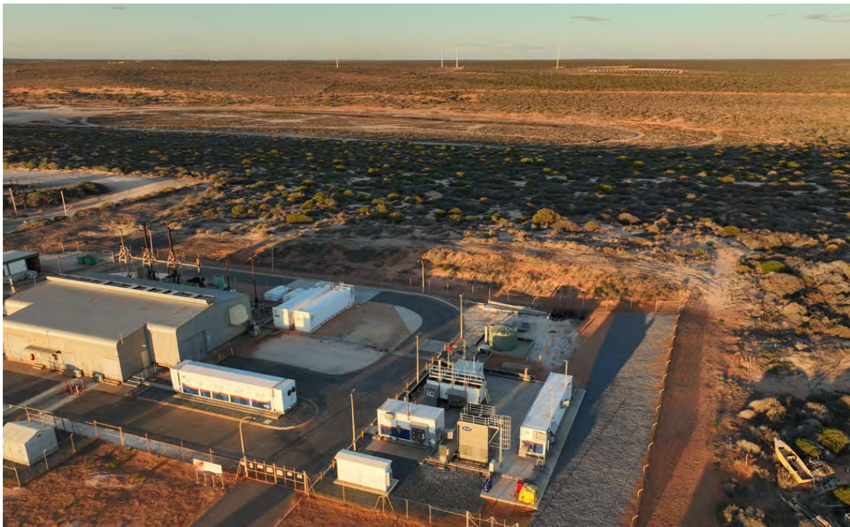
Denham power station and hydrogen plant with the wind and solar farms at the horizon.
