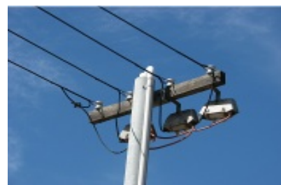
Figure 17: Commercial 3 phase 4 single core connection
