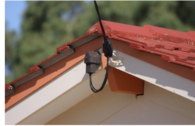
Figure 14: Standard overhead connection and PoA
