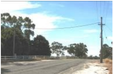
Figure 15: Domestic aerial service cable connection (3 phase)
