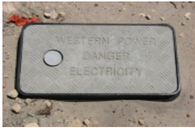
Figure 8: Below ground UMS pit
