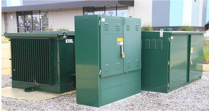
Figure 56: Non modular package (cluster) substation arrangement
