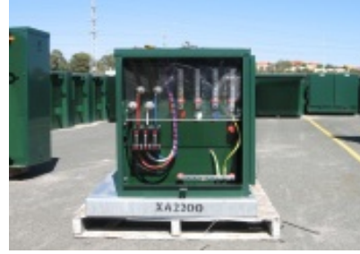
Figure 13: Rural/SPUD transformer supply (1 phase)
