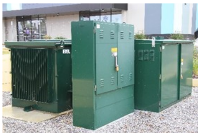
Figure 12: Non MPS (cluster) substation
