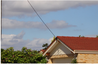
Figure 14: Standard overhead connection and PoA
