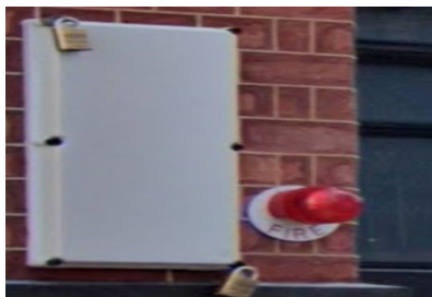
Figure 10: 100A/200A cut out box
