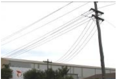
Figure 17: Commercial 3 phase 4 single core connection
