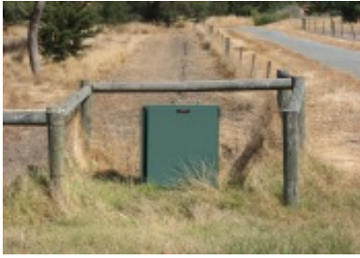
Figure 13: Rural/SPUD transformer supply (1 phase)
