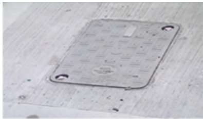
Figure 9: Below ground network pit
