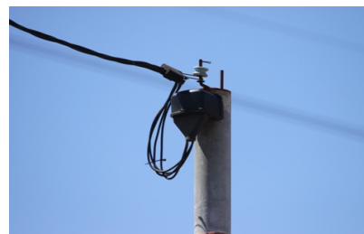
Figure 15: Domestic aerial service cable connection (3 phase)
