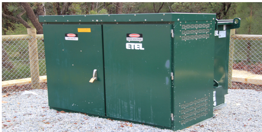
Figure 55: Modular package substation
