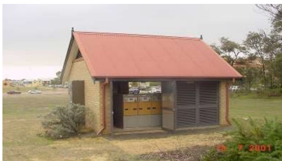
Figure 3 – Brick enclosure Substation.
